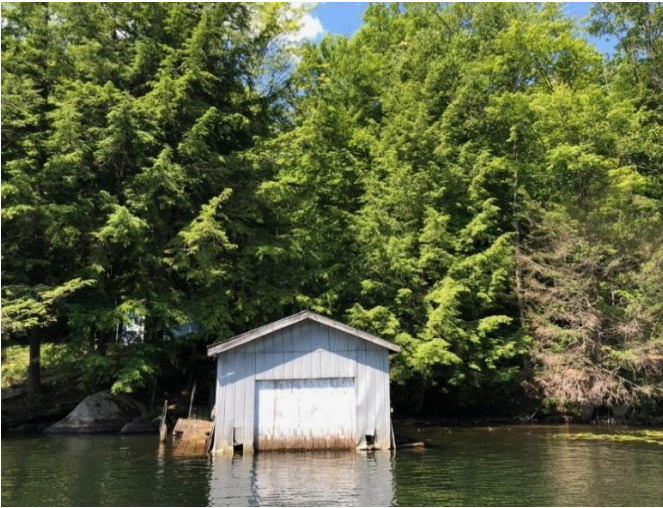
Figure 1 View of existing boathouse from the water.
