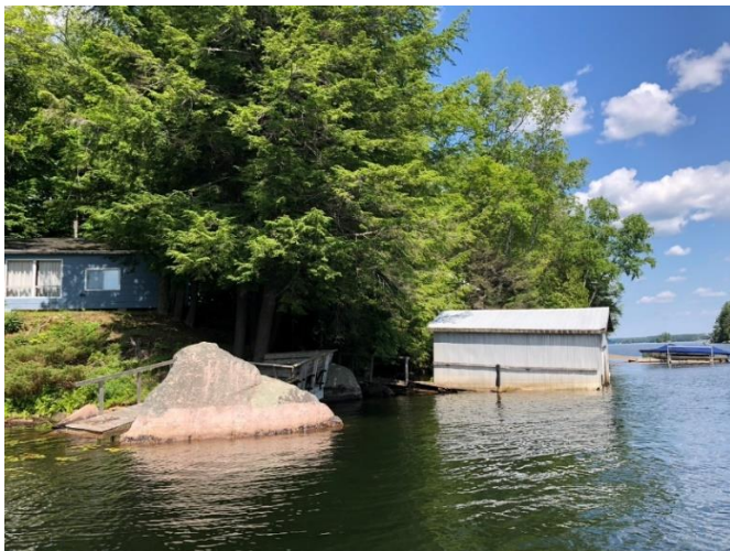
Figure 3 Side profile of the existing boathouse.
